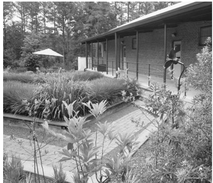
Constructed wetlands in Chatham County, NC
